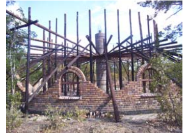
Construction of the Community Conservation and Education Centre
